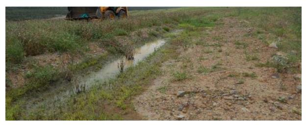
Figure 5-1: Example from the Bowen Basin settlement in a contour drain leading to ponding and development of low points in the contour drain embankment
