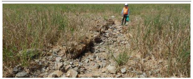
Figure 5-2: Example from the Bowen Basin of minor gully erosion from a contour drain due to settlement of the landform and overtopping
